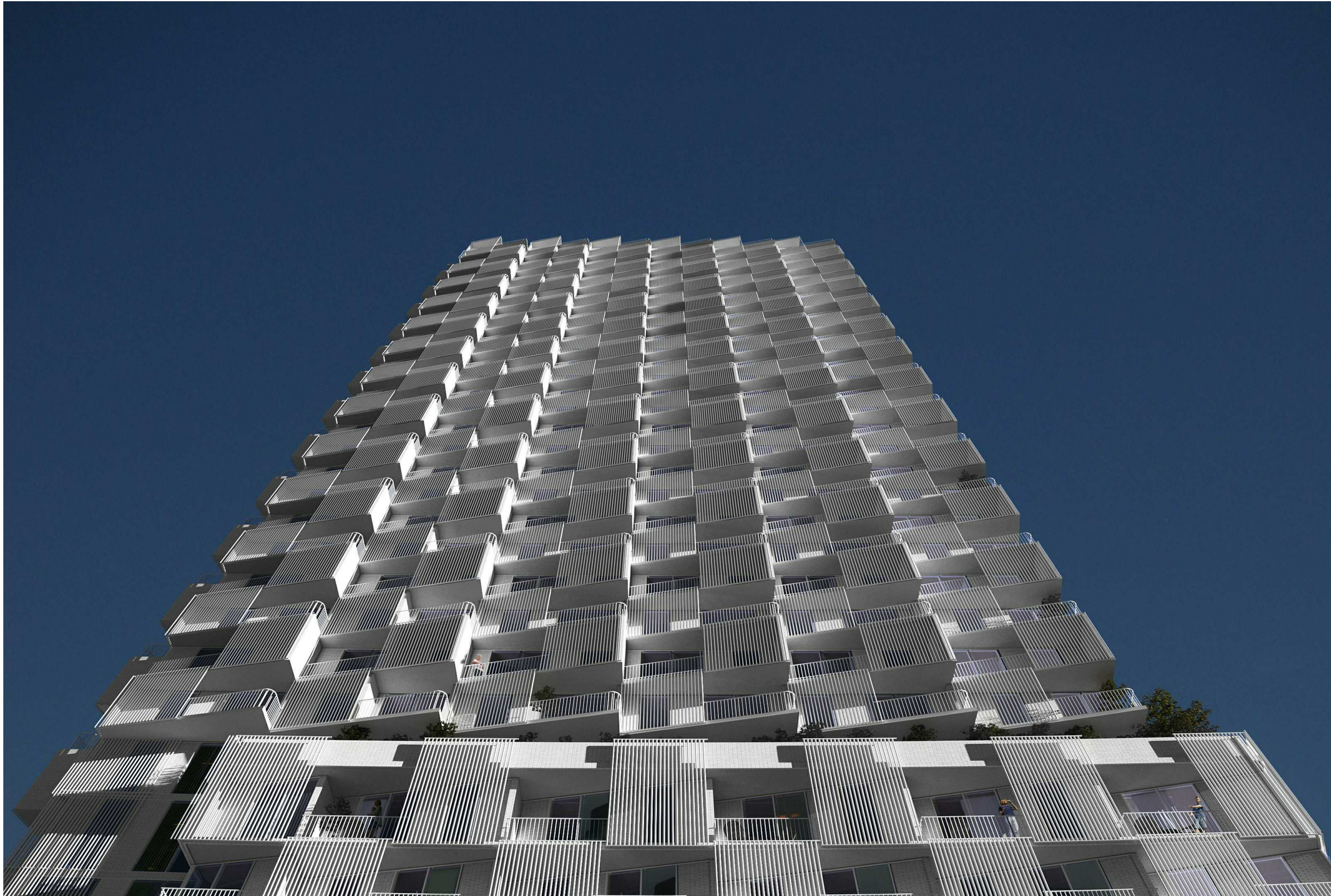
LOOKING UP AT SOUTH SIDE OF BUILDING ALONG EGLINTON AVENUE WEST
