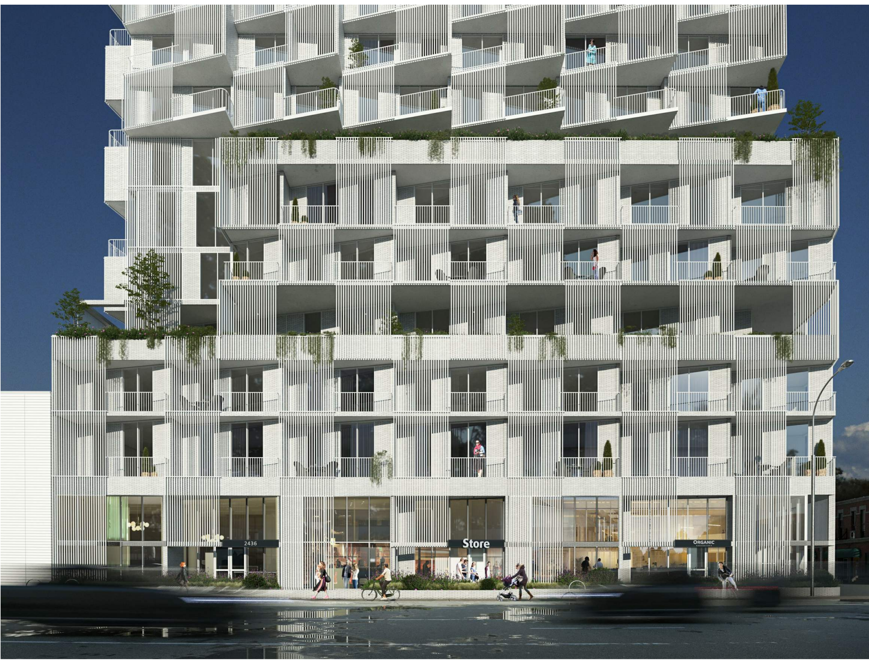
SOUTH ELEVATION VIEW
