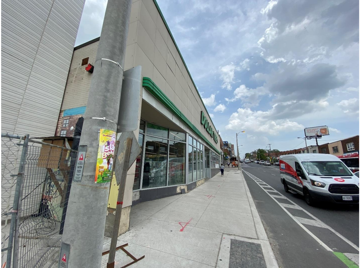
Figure 11. Subject property (facing northeast).
