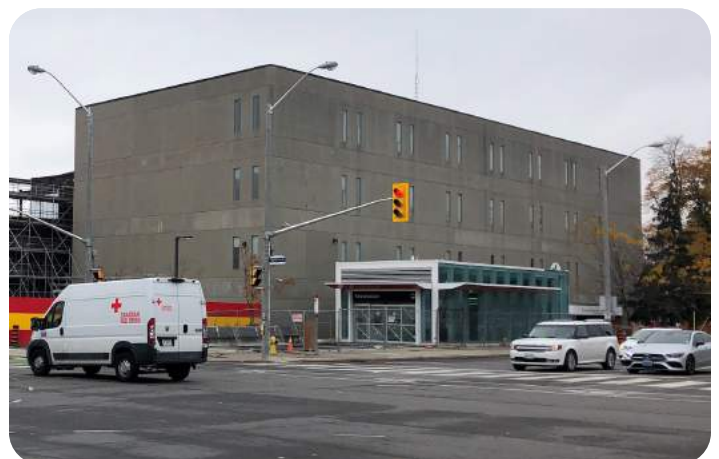
Keelesdale LRT Station (2 Trethewey Drive)
