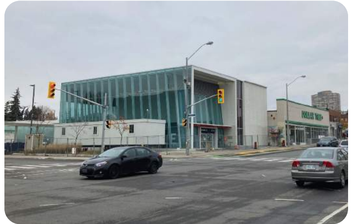
Keelesdale LRT Station (2660 Eglinton Avenue West)
