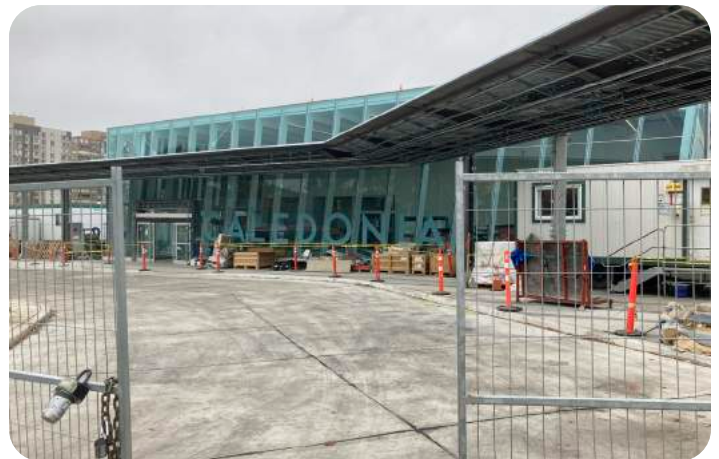
Keelesdale LRT Bus Loop Station (2660 Eglinton Avenue West).
