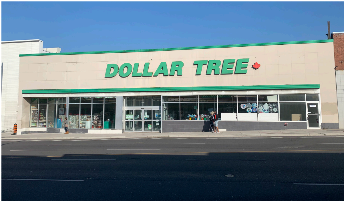
Figure 6. South elevation of 2654 Eglinton Avenue West (ERA, 2022).
