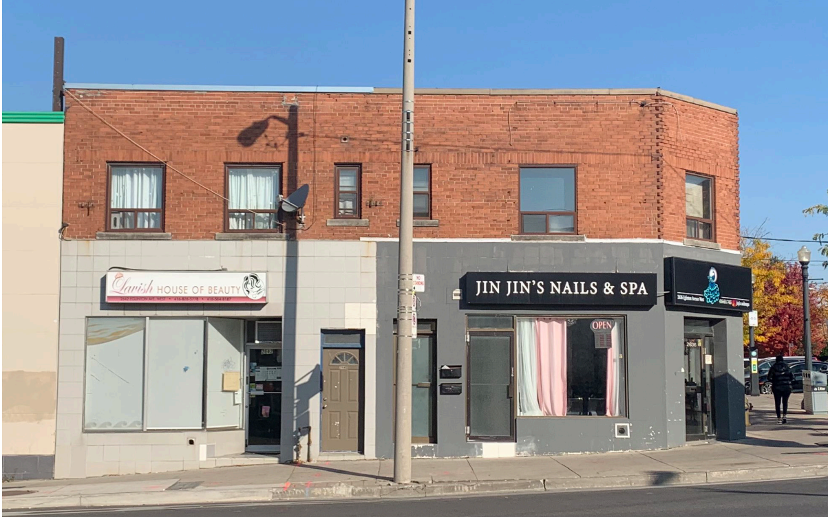
Figure 7. South elevation of 2636-2640 Eglinton Avenue West (ERA, 2022).
