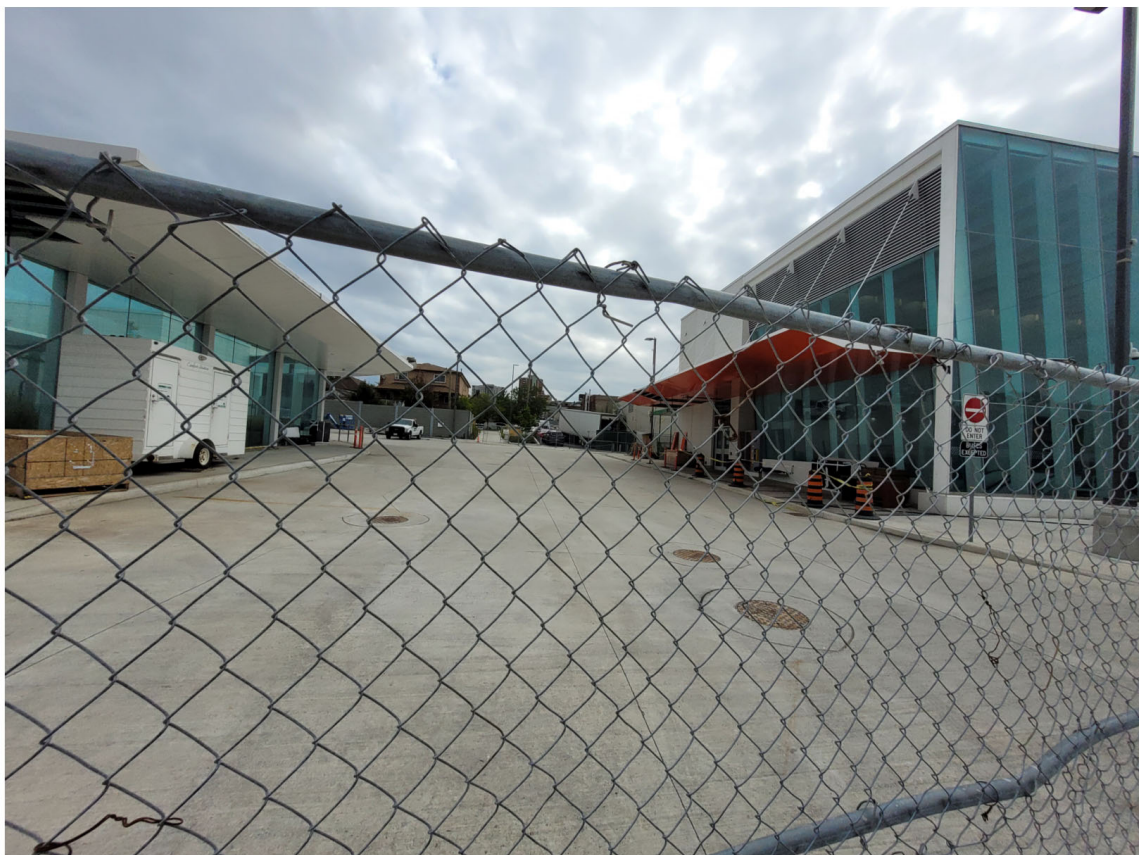
Northwest Corner of Keelesdale Station
