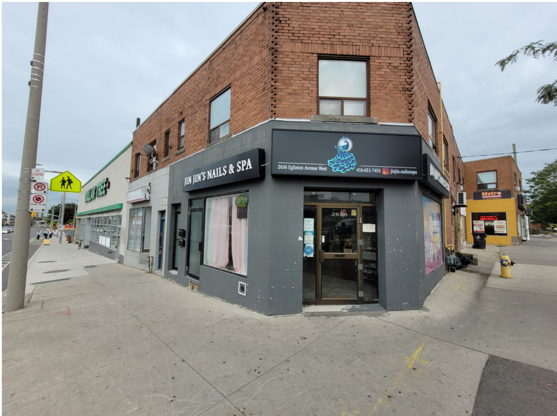
Southeast Corner of 2636 Eglinton Ave W
